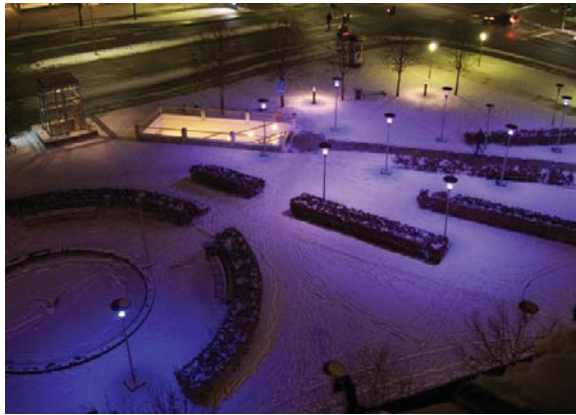
Figure 2: Overview of the Kennedy square with the 16 lamps, seen from the position of the thermal cameras.
